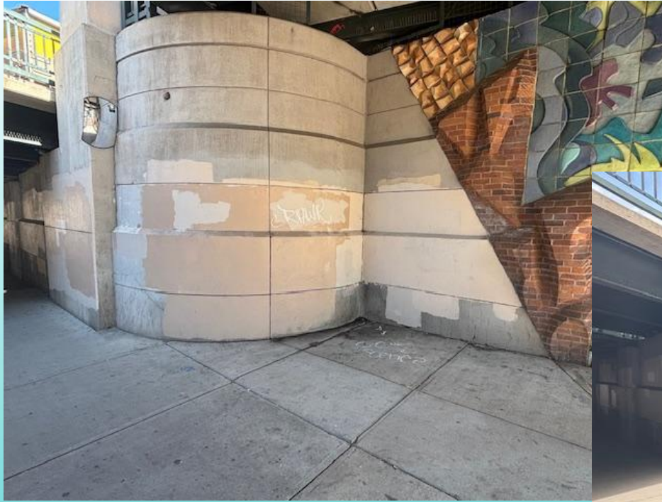
Curved Wall 15th St. Under Train Overpass Bridge Color and Paint Test
